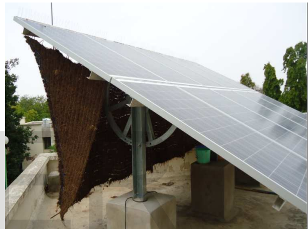
Fig. 1: Khas Tatti for rendering cooling effect on the PV Panel
